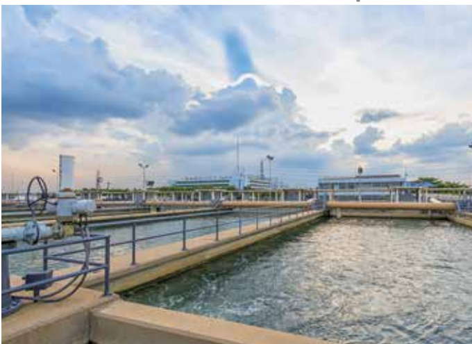
Waste Treatment Plants - Station d'épuration
